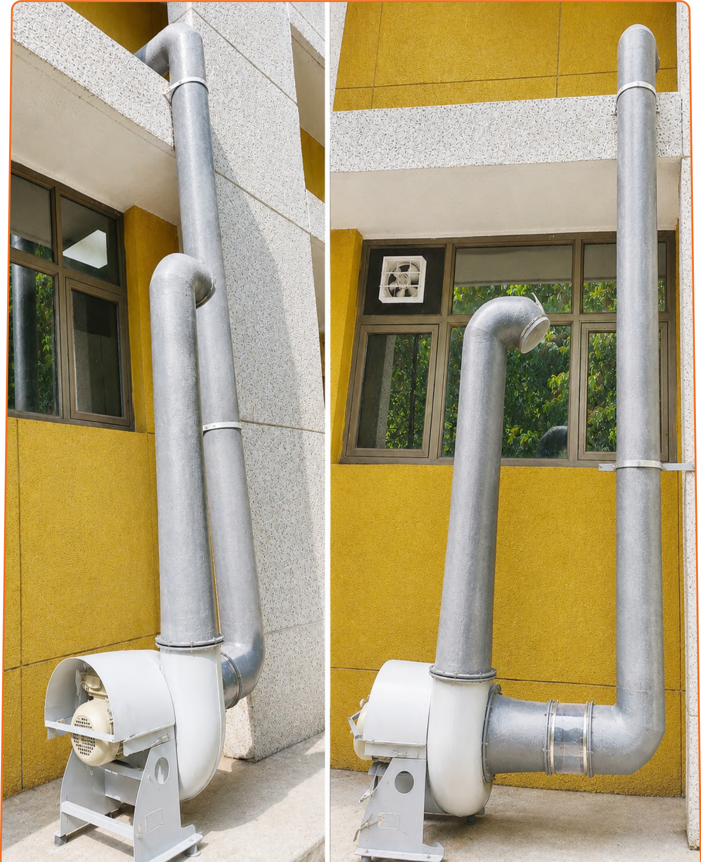
SITE INSTALLATION OF PP BLOWER AND PP/FRP DUCTING
